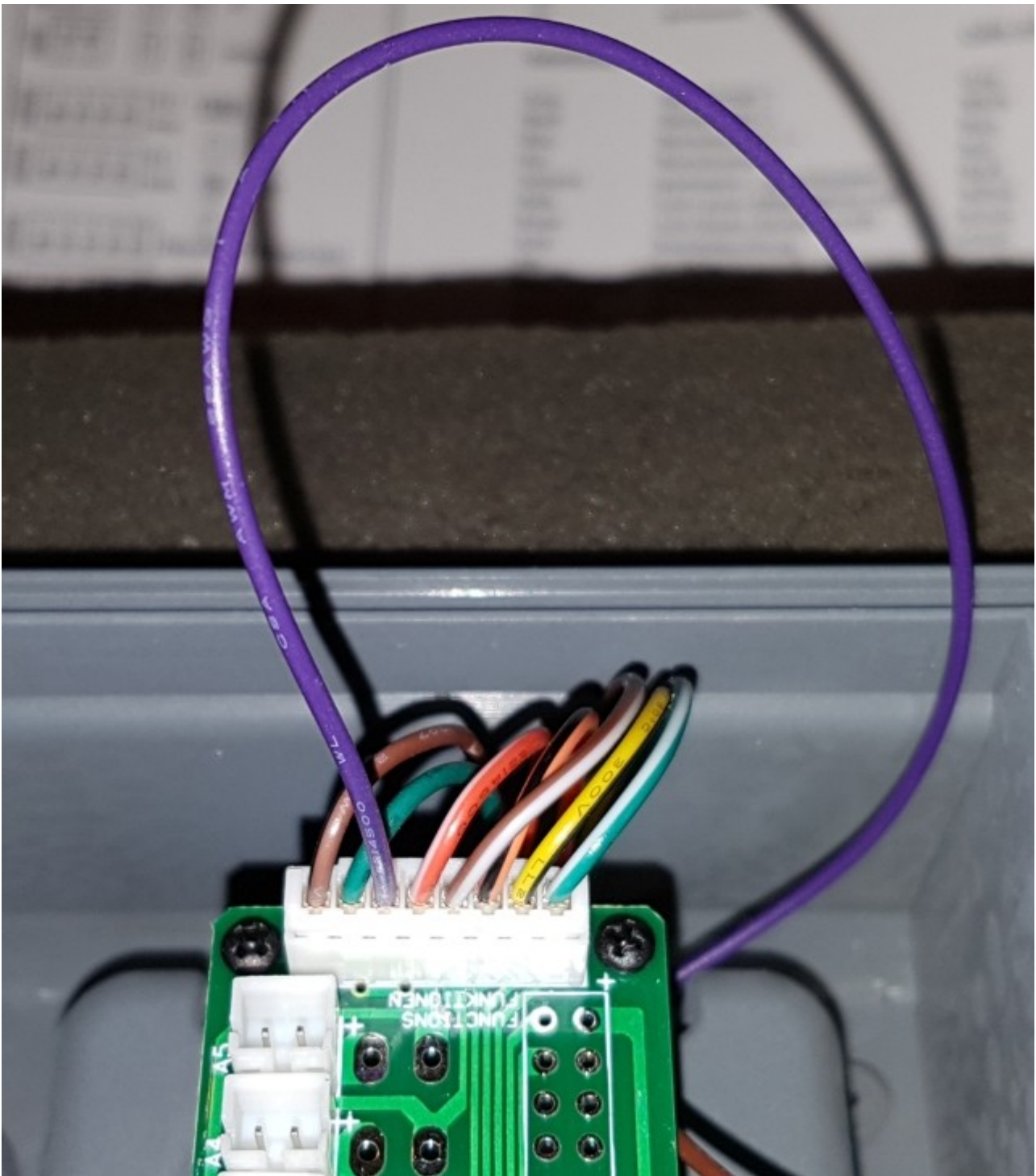
Picture 9: Prepare wire for high beam.
